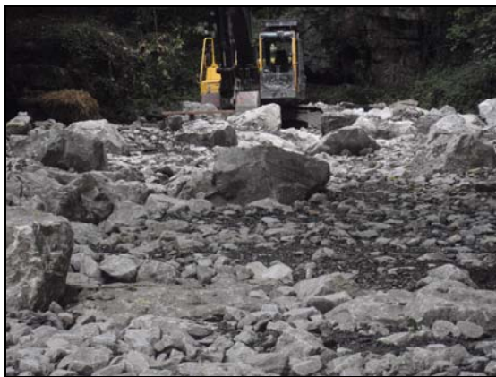
Title: Rocky ramp fish pass construction
