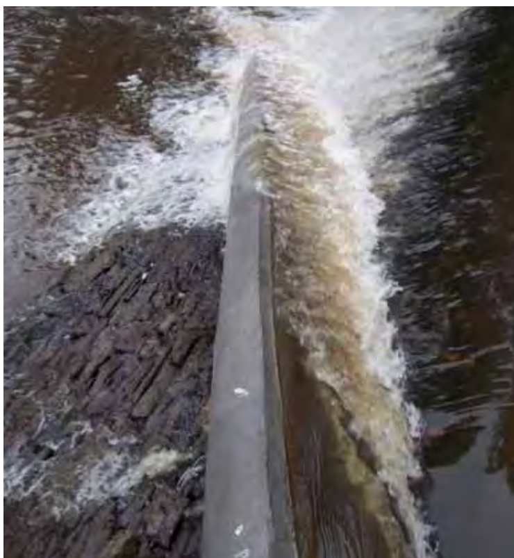
A baulk fish pass at Hunton on the River Arrow. This is one of several on the Arrow and a very cost effective way of restoring fish access on rivers with many weirs.
